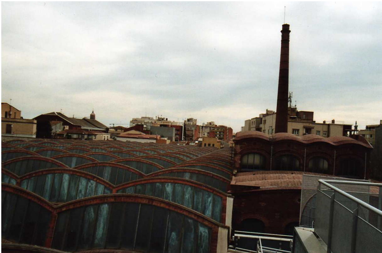
Figure 1 Building of the famous textile industry in Terrassa now turned into a museum
