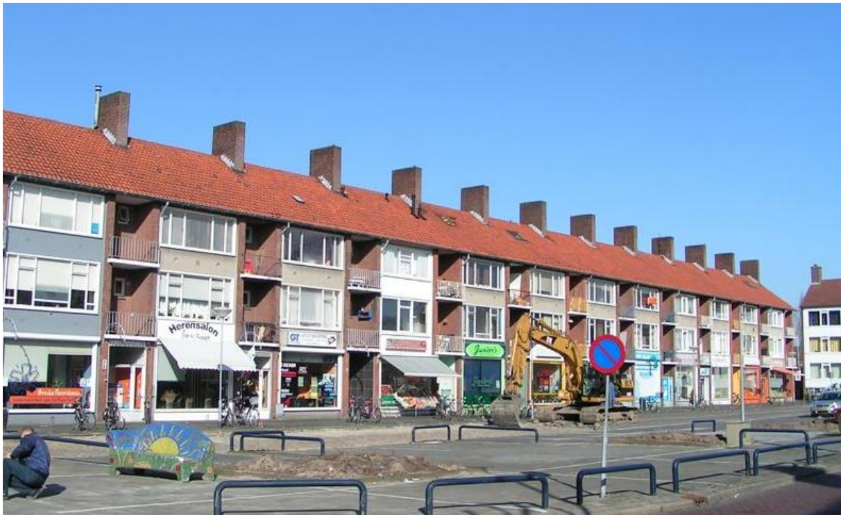
Figure 15 The long stretch of the L-shaped Edisonplein, multicultural shopping square under repair
